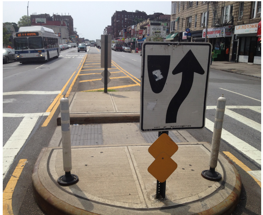
A pedestrian crossing island with accessible-design features including a level, cut-through pedestrian path and detectable warnings in the form of truncated domes, New York, NY. Source: Gerard Soffian
