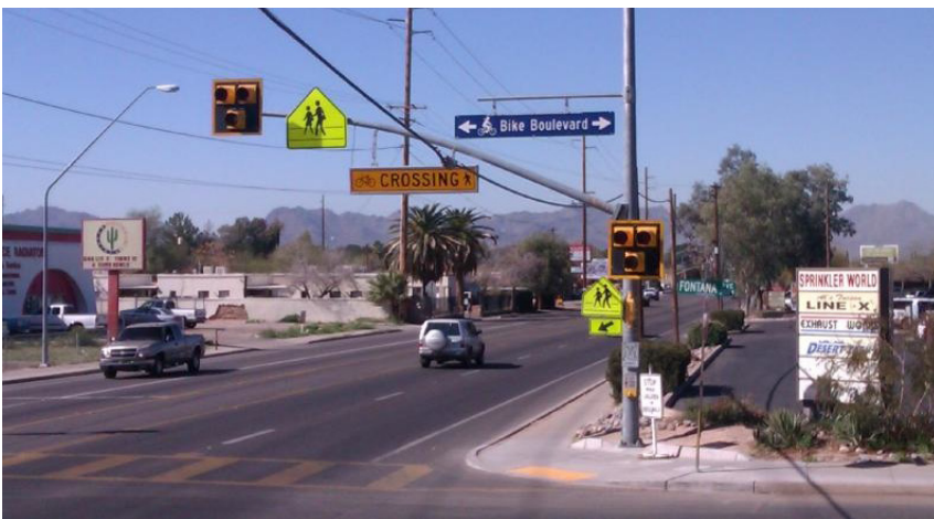
HAWK beacon along Fontana Bike Boulevard at Fort Lowell Road, Tucson, AZ. Source: Tucson Bicycle & Pedestrian Program, City of Tucson
