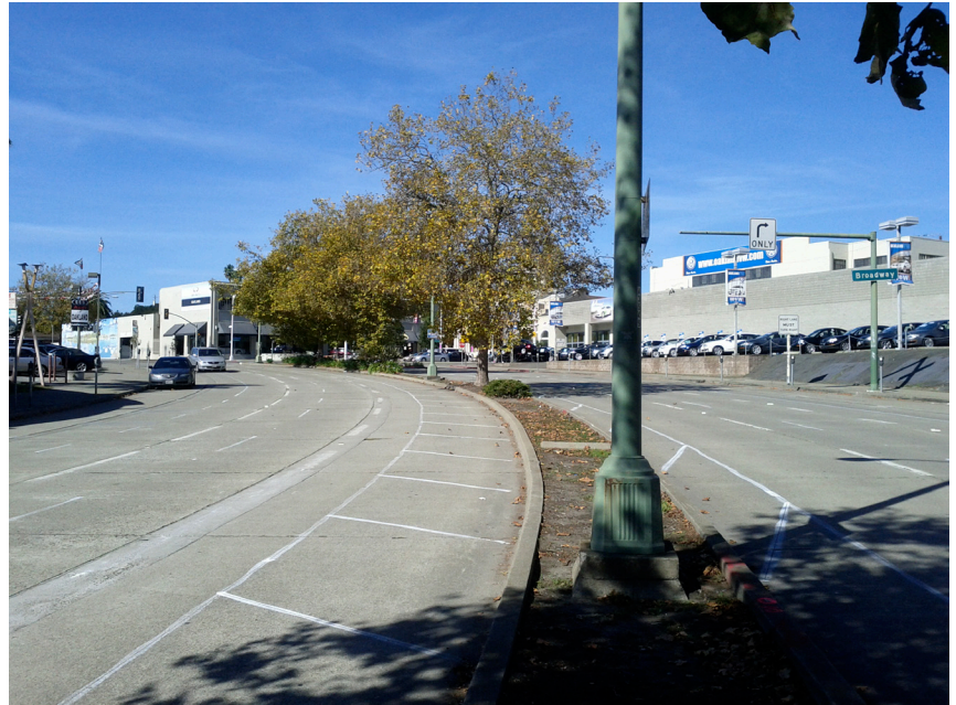
Before restriping narrower travel lanes on 27th Street, in Oakland, CA, workers first sketched out the new street dimensions. Source: Eric Fischer, Flickr
