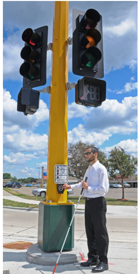
An accessible pedestrian signal with audible tones in Roseville, MN. Source: David R. Gonzalez, MnDOT
