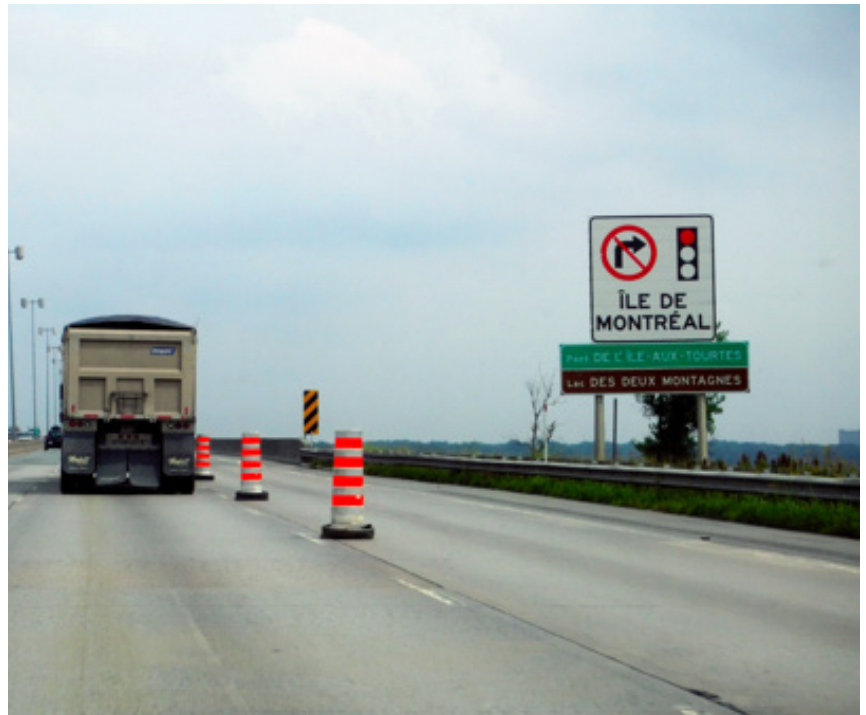
Road signs alert drivers approaching the Island of Montreal that they are entering a zone where no right turns on red are permitted. Source: Vincent Paul Escanlar, betterfredericton.org
