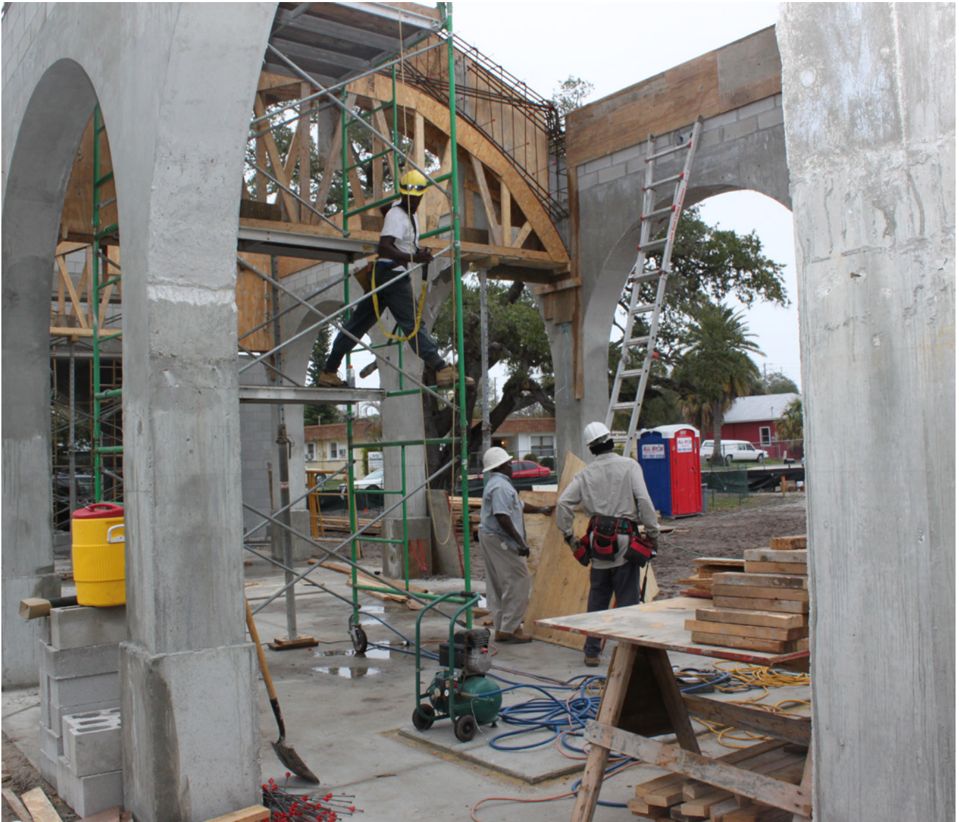
Construction of a transit facility. Flickr: US DOT
